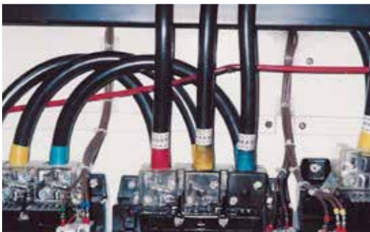
Firetrace detection tubing typical burst hole
